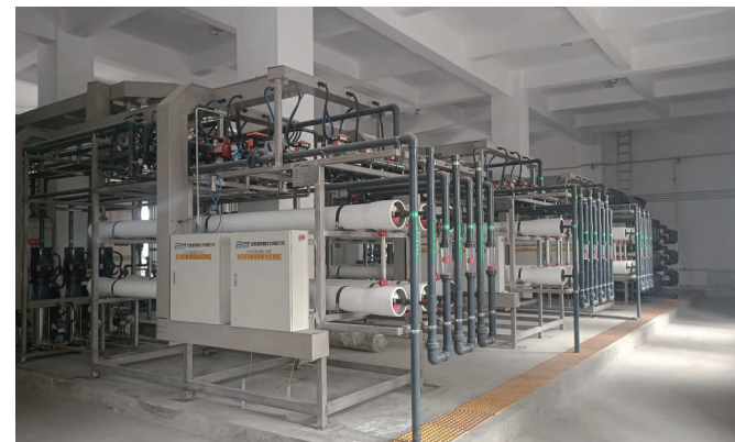
Gansu Power Plant, 2×350MW Unit, 10 m 3 /h Desulfurization Wastewater Zero Liquid Discharge Project
