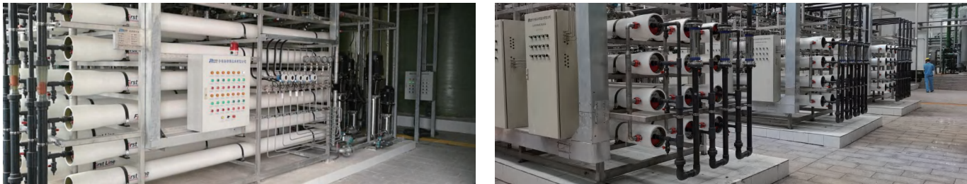
60m³/h Coal Chemical RO Brine and 4 m³/h Crystallization Brine UF+NF – Separation of Monovalent and Divalent Salts
