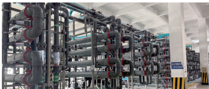
A new 235 m 3 /h reclaimed water reuse unit and a 106 m 3 /h RO brine zero liquid discharge unit were installed for a technology company in Inner Mongolia.
