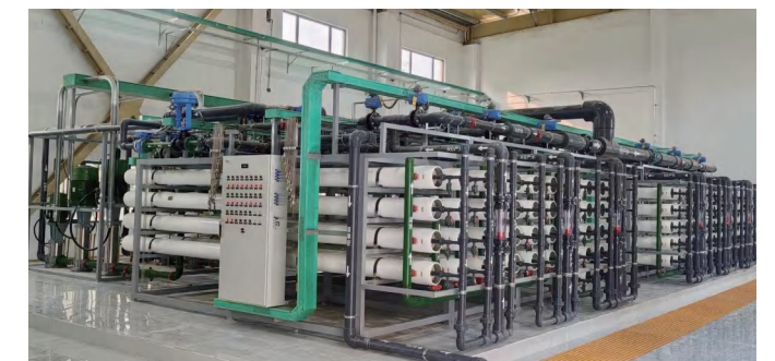
▲ 400 m 3 /h Circulating Water Blowdown Treatment Project for a Photovoltaic Company in Yunnan (Total Water Recovery Rate >90%)
