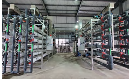
52m³/h Power Plant Cooling Water Blowdown Softening and Hardness Removal Unit
