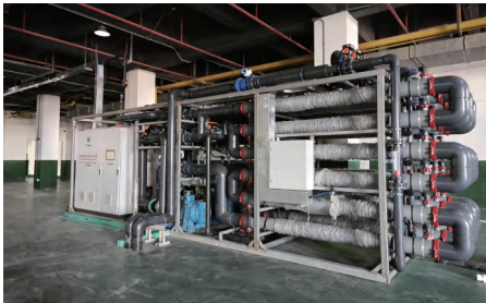
▲ 3000m³/d PCB Wastewater Copper Removal Project
